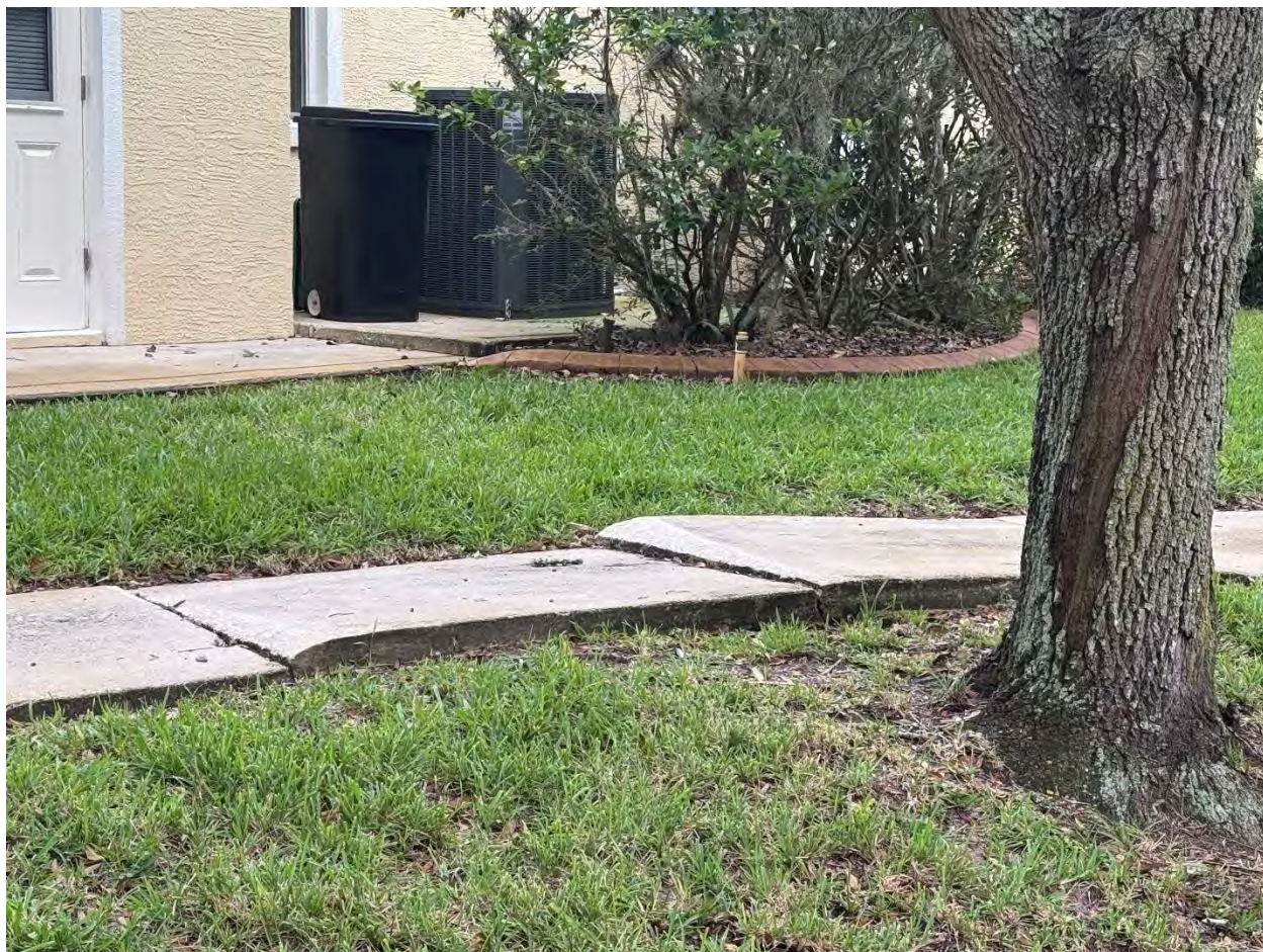
Figure 15 - Sidewalk Bowing
