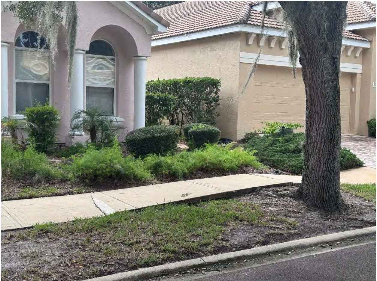
Figure 14 - Sidewalk Bowing
