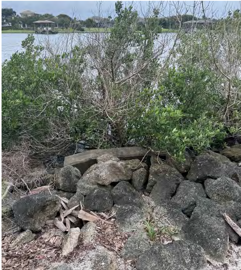
Figure 11 - Pond 5 Outfall into ICW
